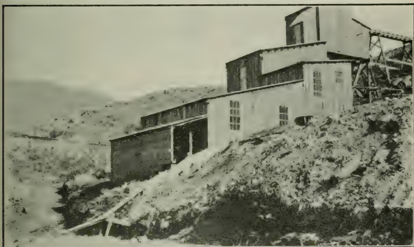
Photo No. 36a. The 50-ton concentrating mill of the California Chrome Company at the Castro Mine, San Luis Obispo.
